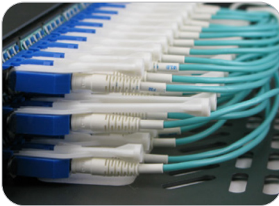
LC uniboot patch leads allow maximum access to the patching environment.
