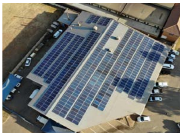
Installation of solar panels at a Zalawi Whitehorse site
