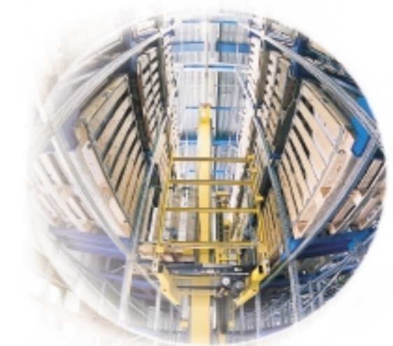
FULLY AUTOMATED WAREHOUSE
