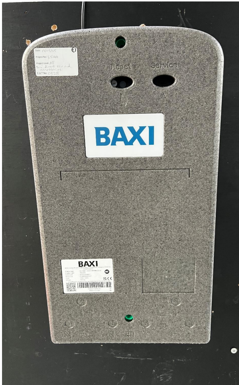
Figure 20 - HIU with Outer Case Fitted
