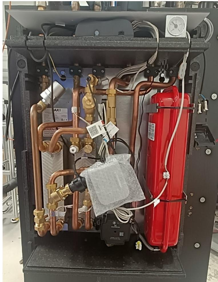
Figure 21 - HIU with Outer Case Removed
