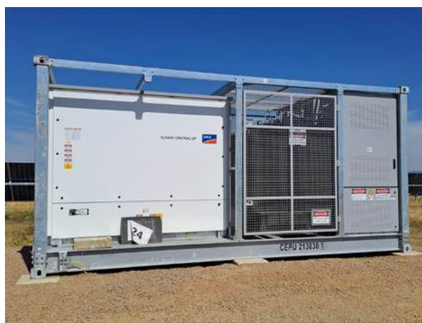
Plate 2 – PCU at Glenrowan Solar Project (source: Pacific Partnerships, 2025)
