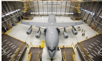
RAAF Base Amberley Multi Role Tanker Transport Facilities, QLD Completed: 2008 $135m
