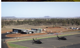
Army Aviation Training Centre Redevelopment, Oakey QLD Completed: 2004 $76.2m
