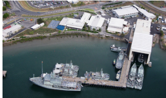
HMAS Cairns Redevelopment, Cairns QLD Completed: 2009 $76.3m
