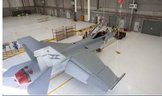
RAAF Base Amberley Australian Super Hornet Facilities, QLD Completed: 2011 $108m
