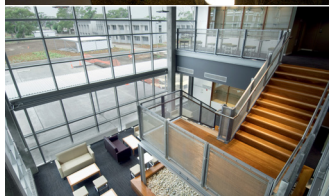
RAAF College Relocation, RAAF Base East Sale VIC and RAAF Base Wagga NSW Completed: 2008 $133m
