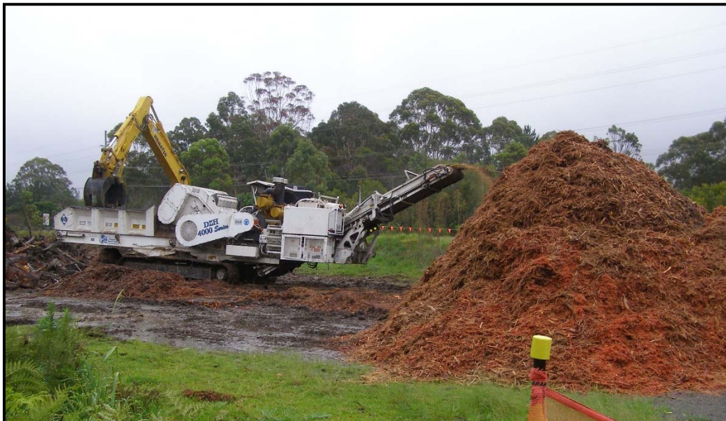
Plate 2: Vegetation mulching activity – mulch should be progressively moved into prepared stockpile areas.
