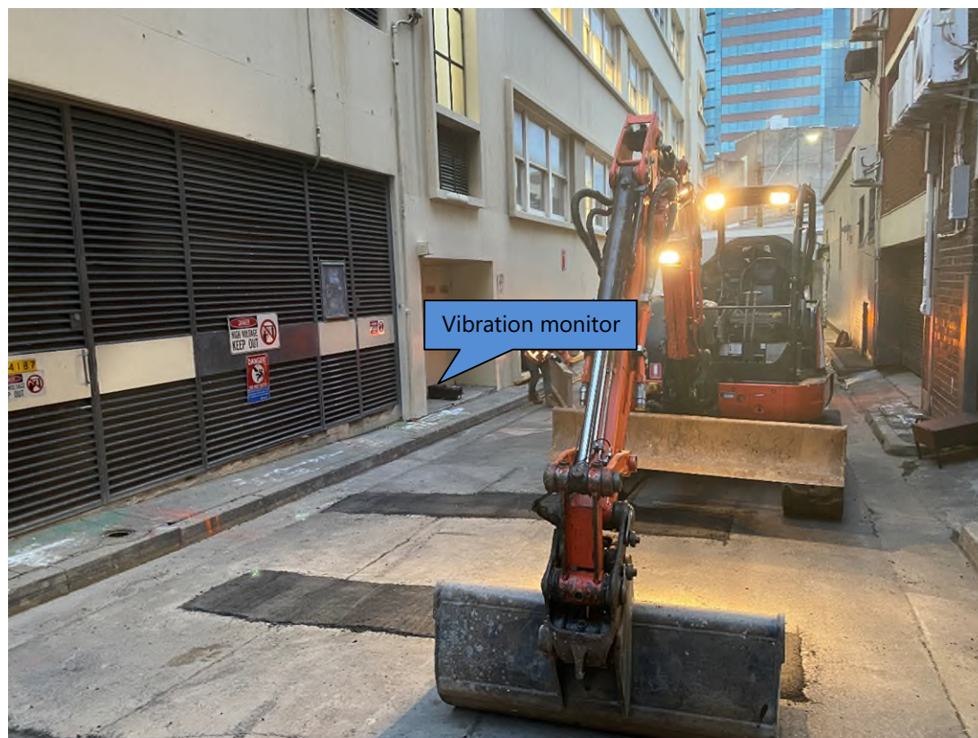
Figure 2-2: Instrumentation set up – Randle Lane unattended vibration monitoring
