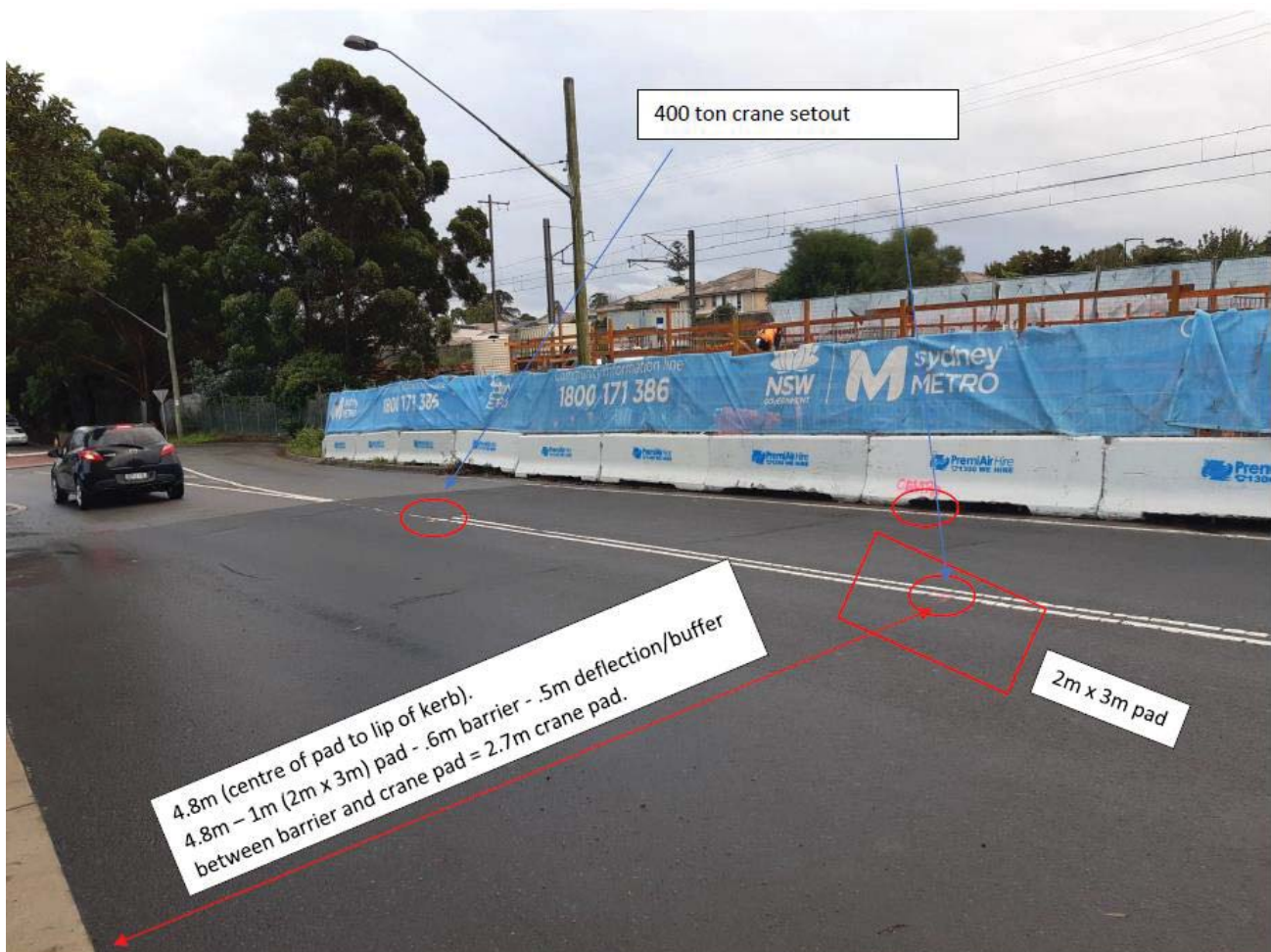
Figure 7. Survey setout to check crane outrigger position to determine constructibility
