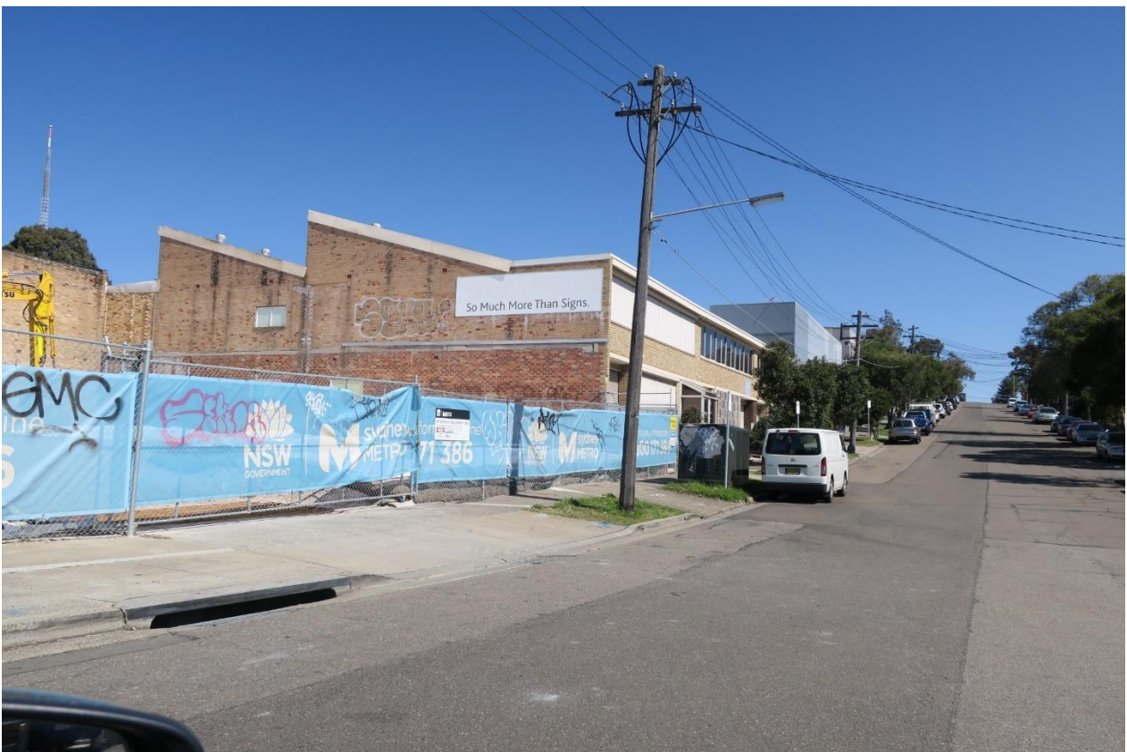
Figure 5 – View from Whiting Street looking towards Clarendon Street on the far end. Artarmon substation site on the left.
