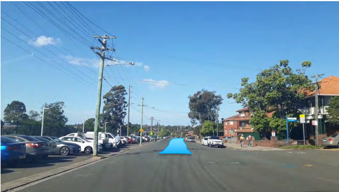
Figure 9 – View at South Parade (looking east) from the intersection of Harold Street. Traffic maintained for both directions.
