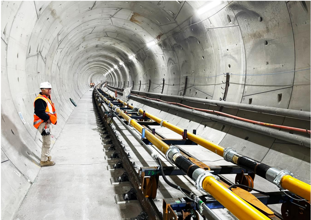
Figure 1. Typical setup of concrete delivery lines in the tunnel
