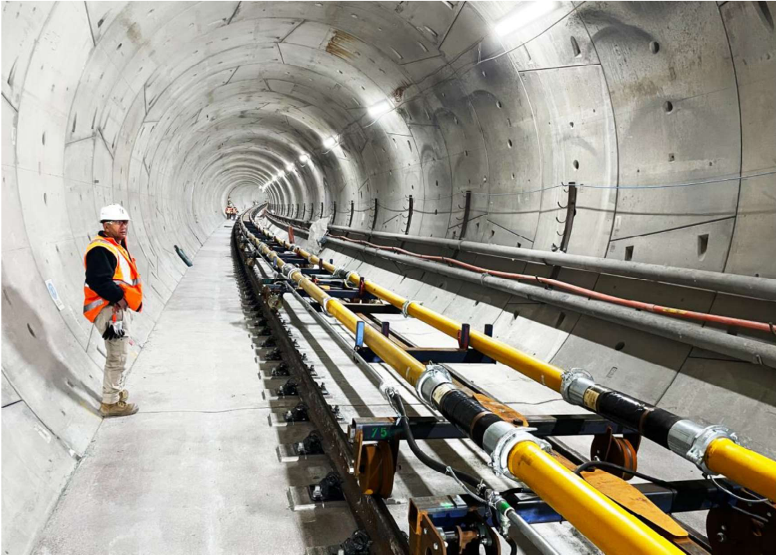
Figure 1. Typical setup of concrete delivery/transfer lines in the tunnel
