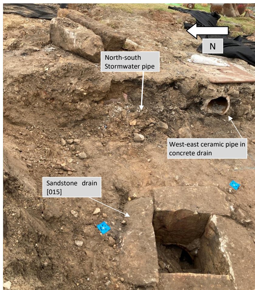
Figure 3.11: Image of the sandstone drain [015] with part of the stormwater drainage pipe in the southeast corner running towards the harbour.
