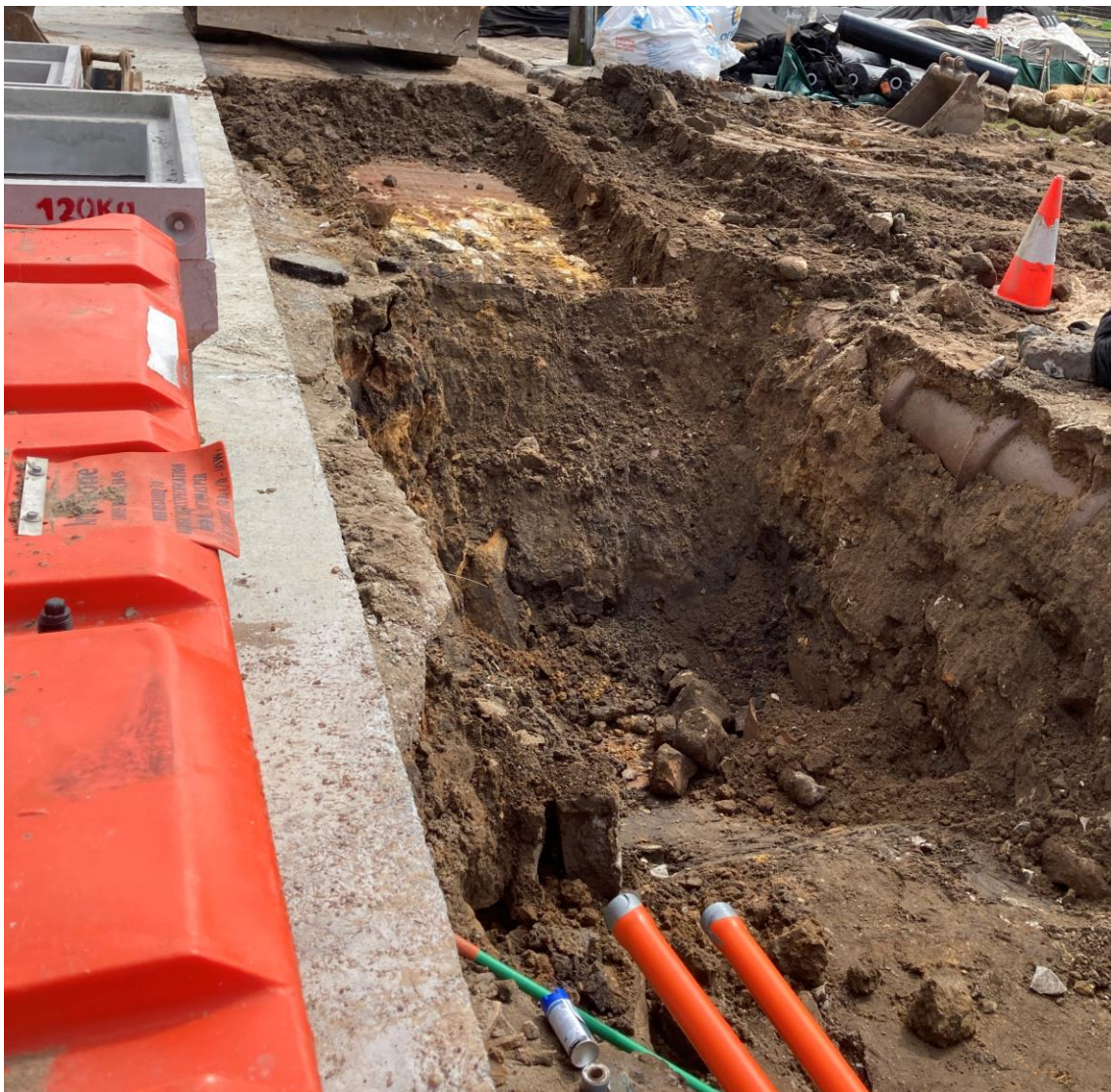
Figure 3.23: Trench for a garden bed in WZ3D showing the exposed bedrock at the top of the trench, a service pipe on the right and the steep natural benching of the bedrock.
