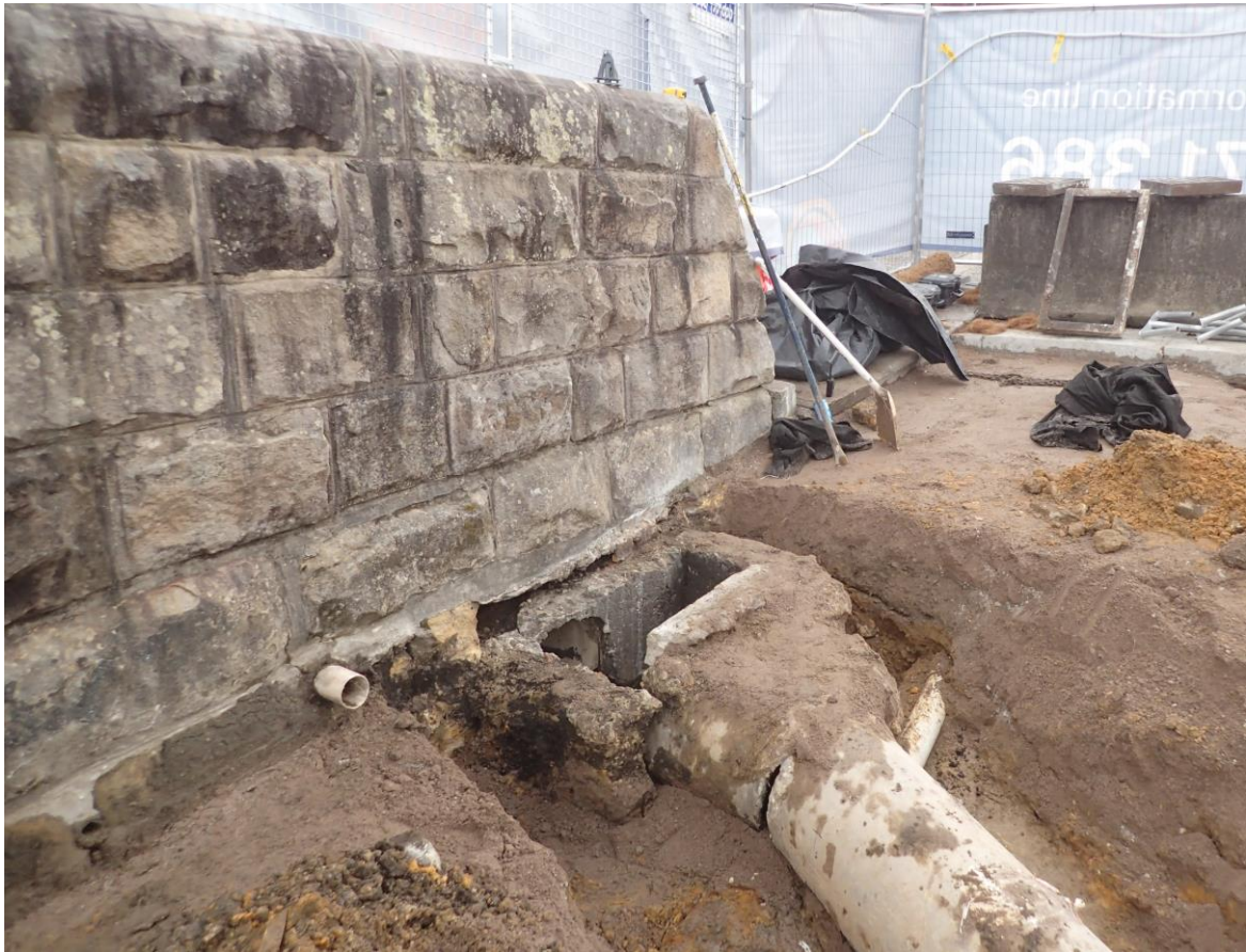
Figure 3.25: The concrete drain and connecting pipe laid under the northern most section of the heritage wall.
