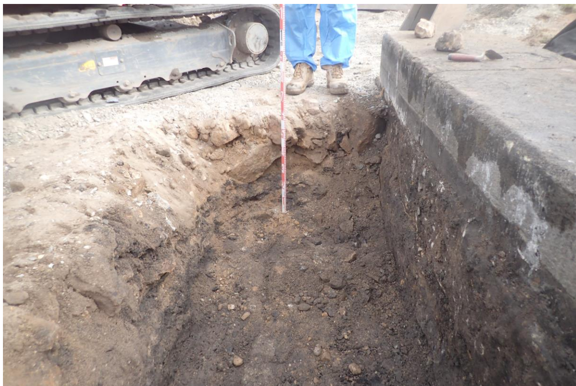
Figure 3.18: The vertical unworked side of the reduced sandstone seawall [328] with the sandstone kerbing above.
