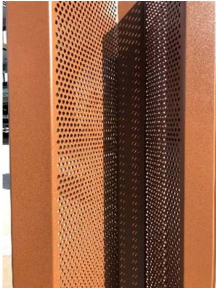
Figure 3 – Finish Type 1 - Folded and perforated pre weathered -Weathering Steel (Corten)
