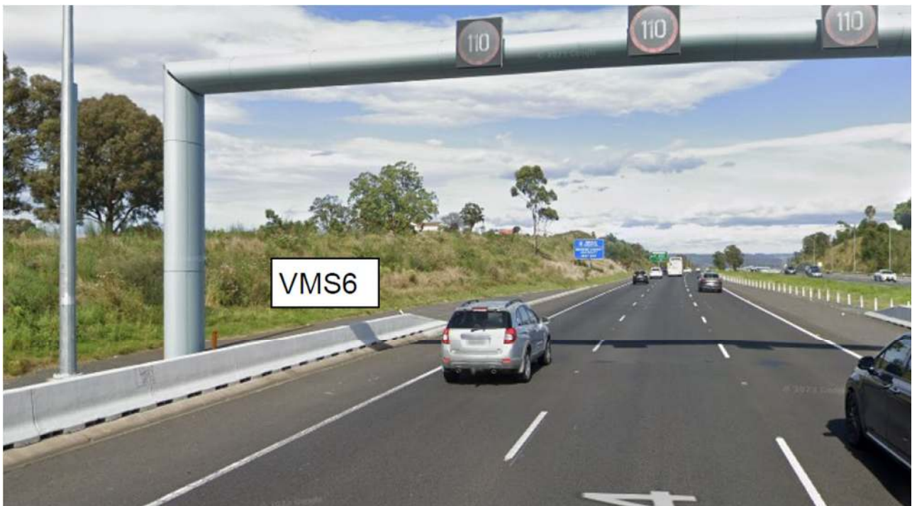
Figure 1748: VMS6 M4 Westbound in METS bay
