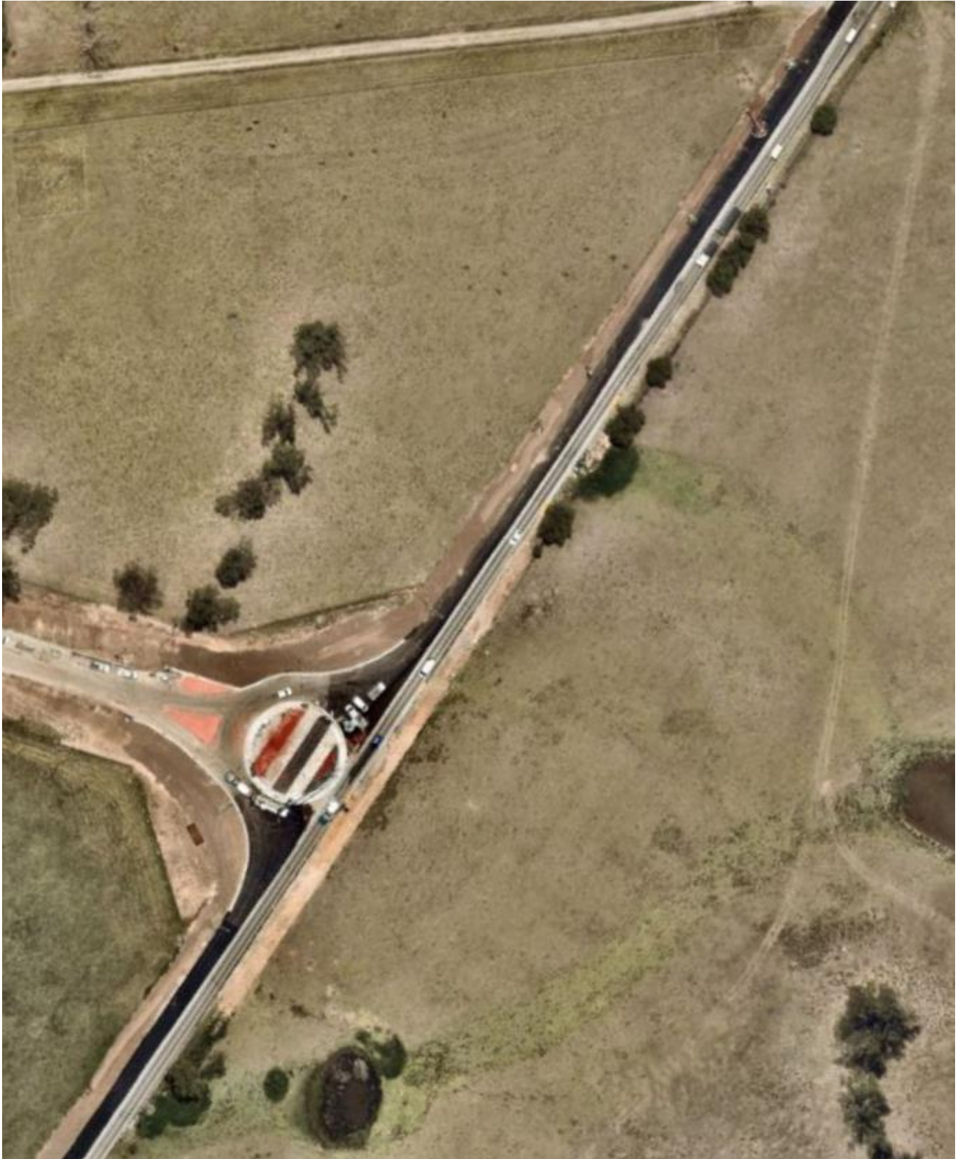
Figure 6: Roundabout work site (Nearmap 17 Nov 23)
