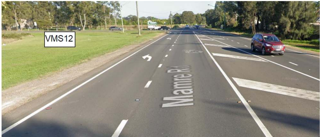
Figure 2021 : VMS12 Mamre Road south of Luddenham Road facing northbound traffic
