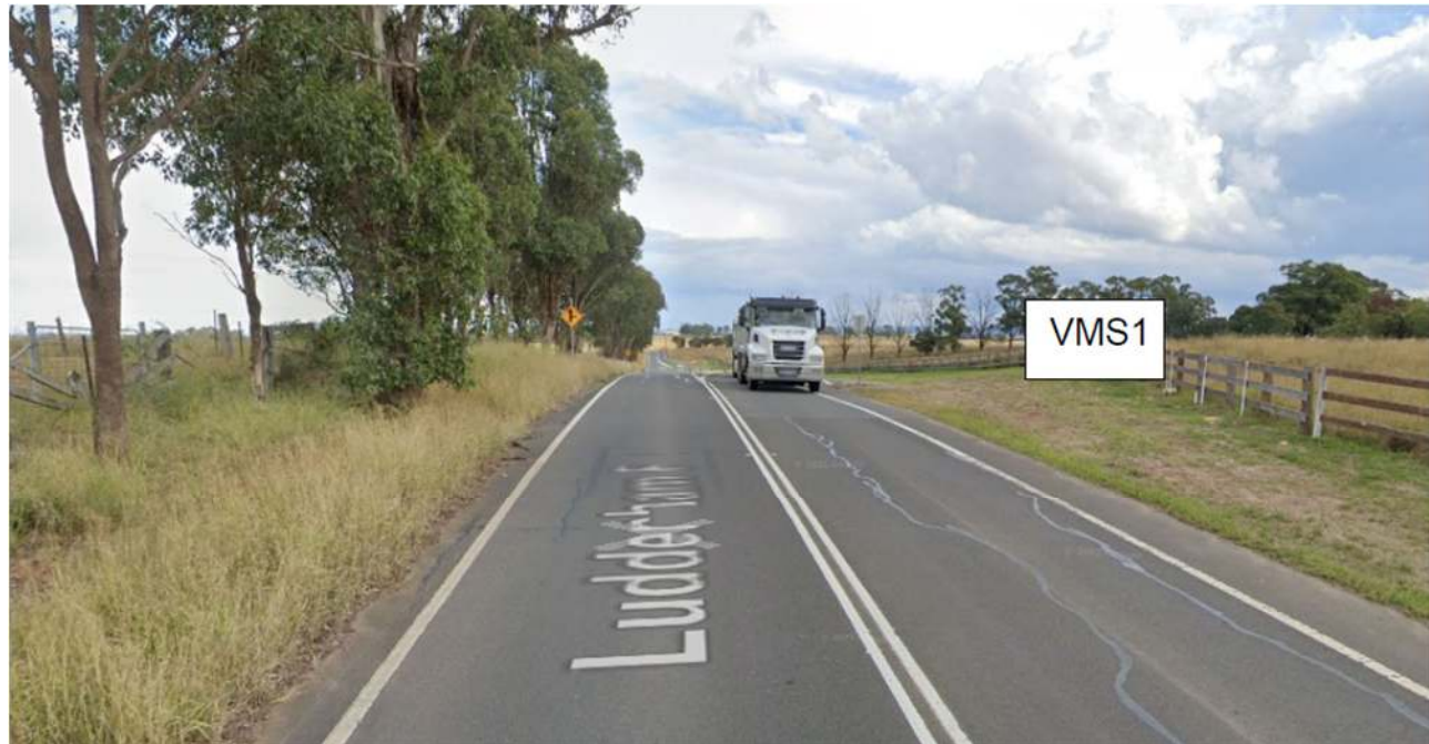
Figure 1445: VMS 1 facing southbound traffic on Luddenham Road
