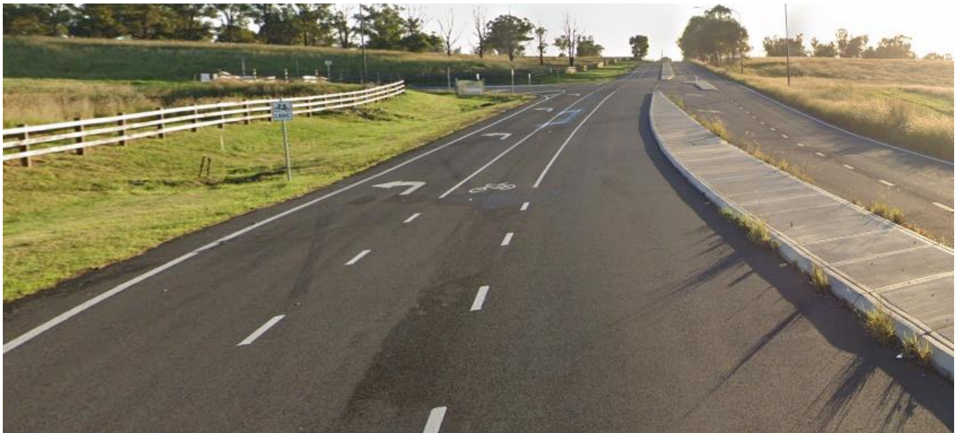
Figure 10: On road cycle facility at Gate 4
