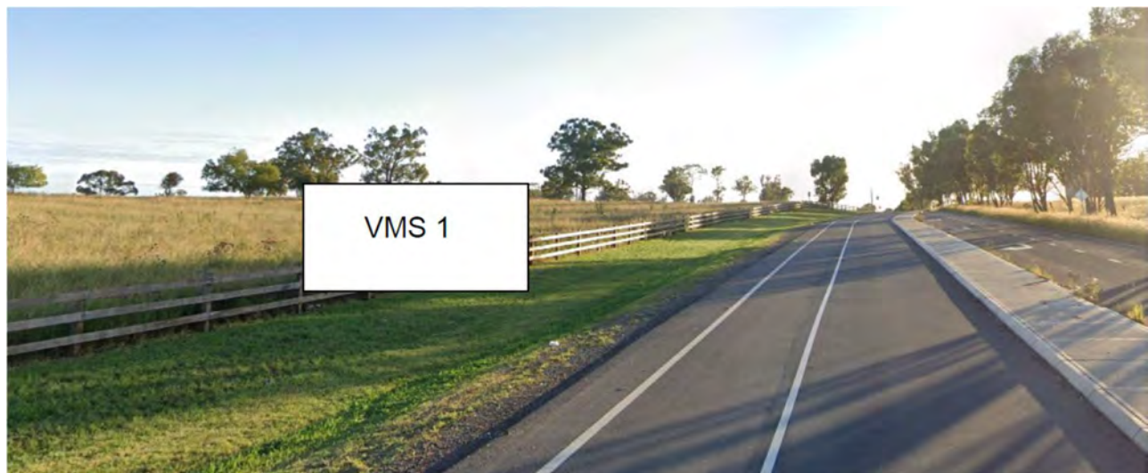
Figure 15: VMS 1 for northbound traffic
