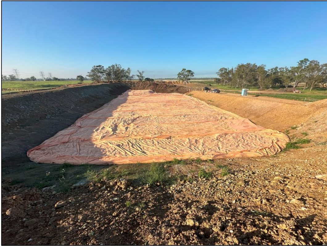
Site Photograph 1. Top of PS105 containment cell, following placement of mastaTEX Orange Hi Vis Geotextile Warning Layer (facing east), as observed 1 February 2024.
