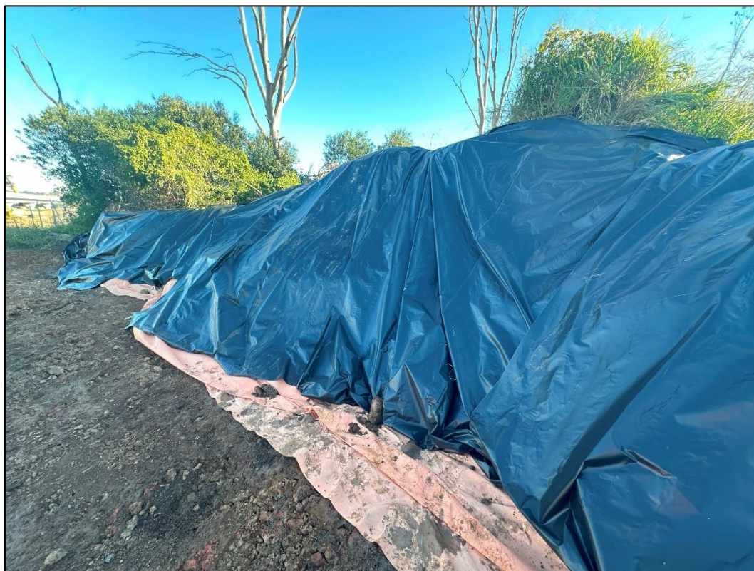
Photograph 2 View of the Subject Area following being covered with geofab and black plastic, as viewed facing west, as observed 28 May 2024.
