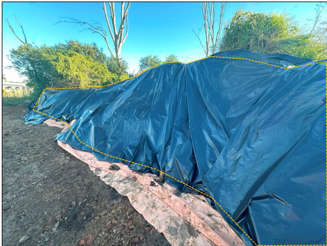
Site Photograph 7.1.3 View of the western wall following installation of the geofabric layer, as observed 28 May 2024 viewed facing south-west.
