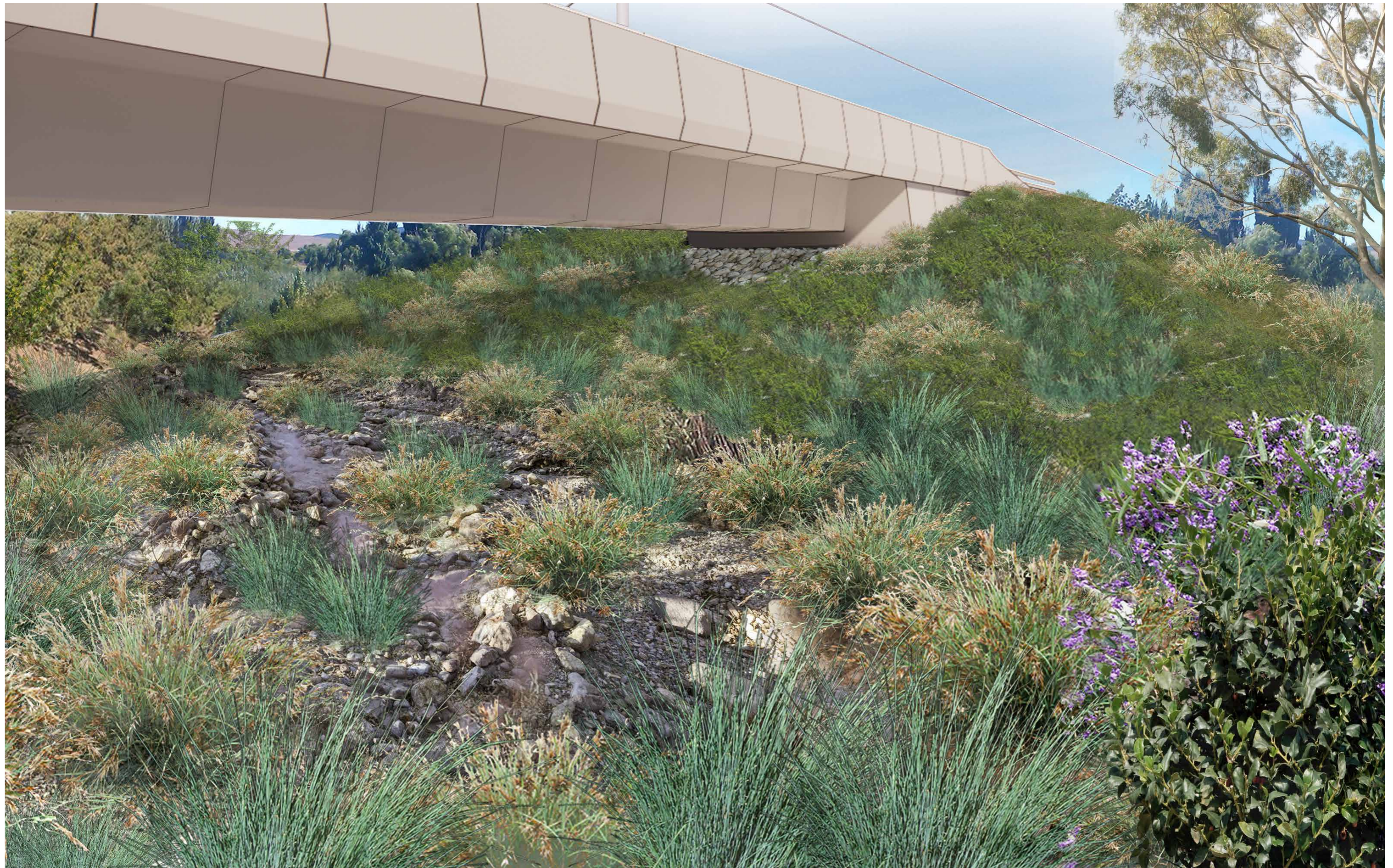
Figure 29 - Viaduct and Embankment
