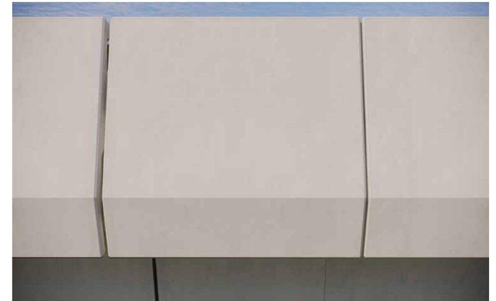
Figure 22 - Parapet Joints
