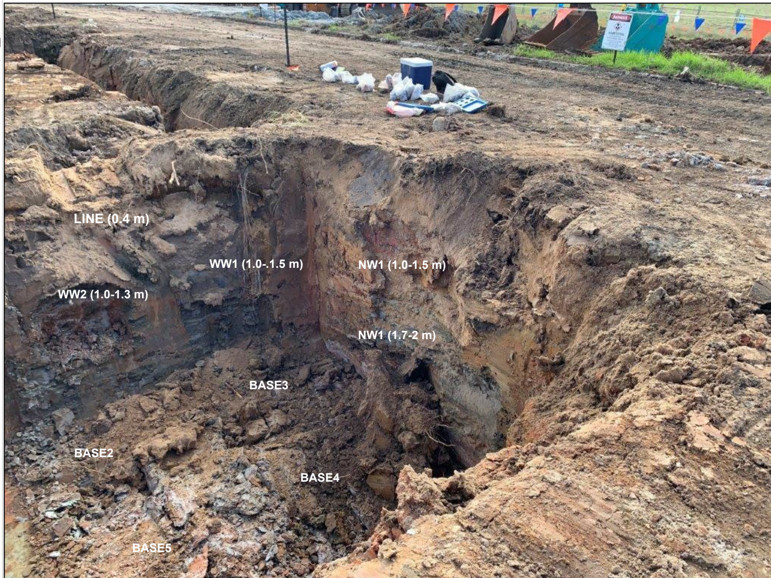
Photograph 3 – North Wall, partial west wall and partial base (base samples 2.4 m)
