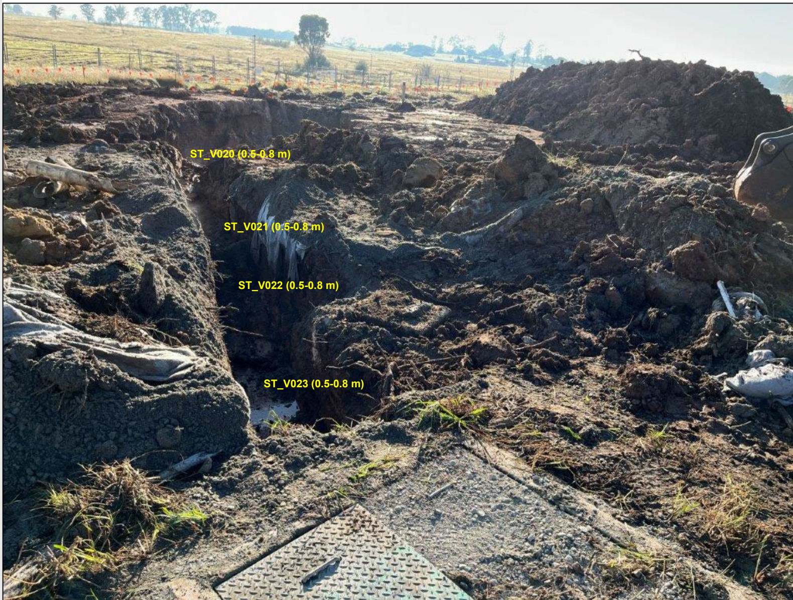
Photograph 4 – Associated pipework trench
