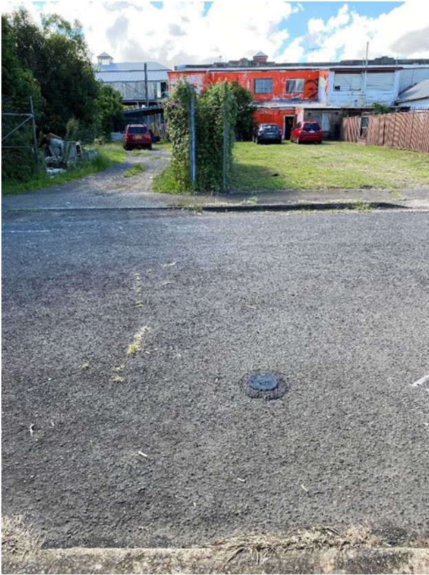
Rear of 1-7 Queens Street (Former Dry Cleaners); photograph taken from West Lane
