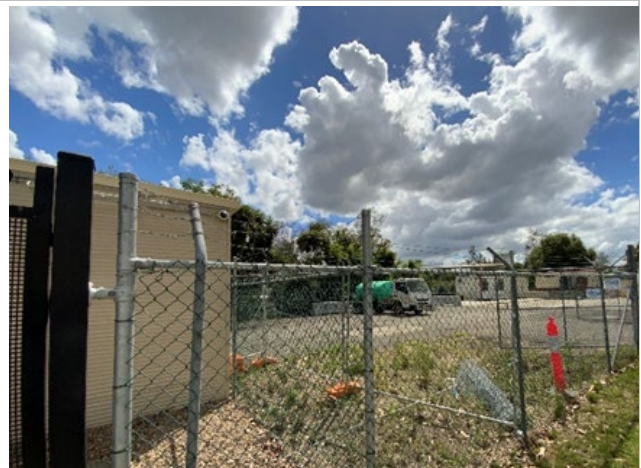
1-2 Station Street (bus drivers compound)
