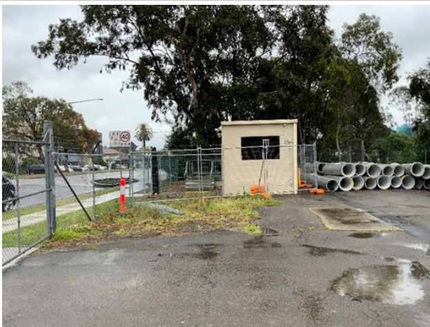
1-2 Station Street (bus drivers compound)
