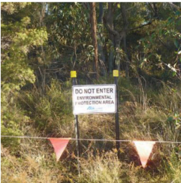
Figure 3: Example of Environmentally Sensitive Area exclusion fencing and signage (Source: TR&T 2010)
