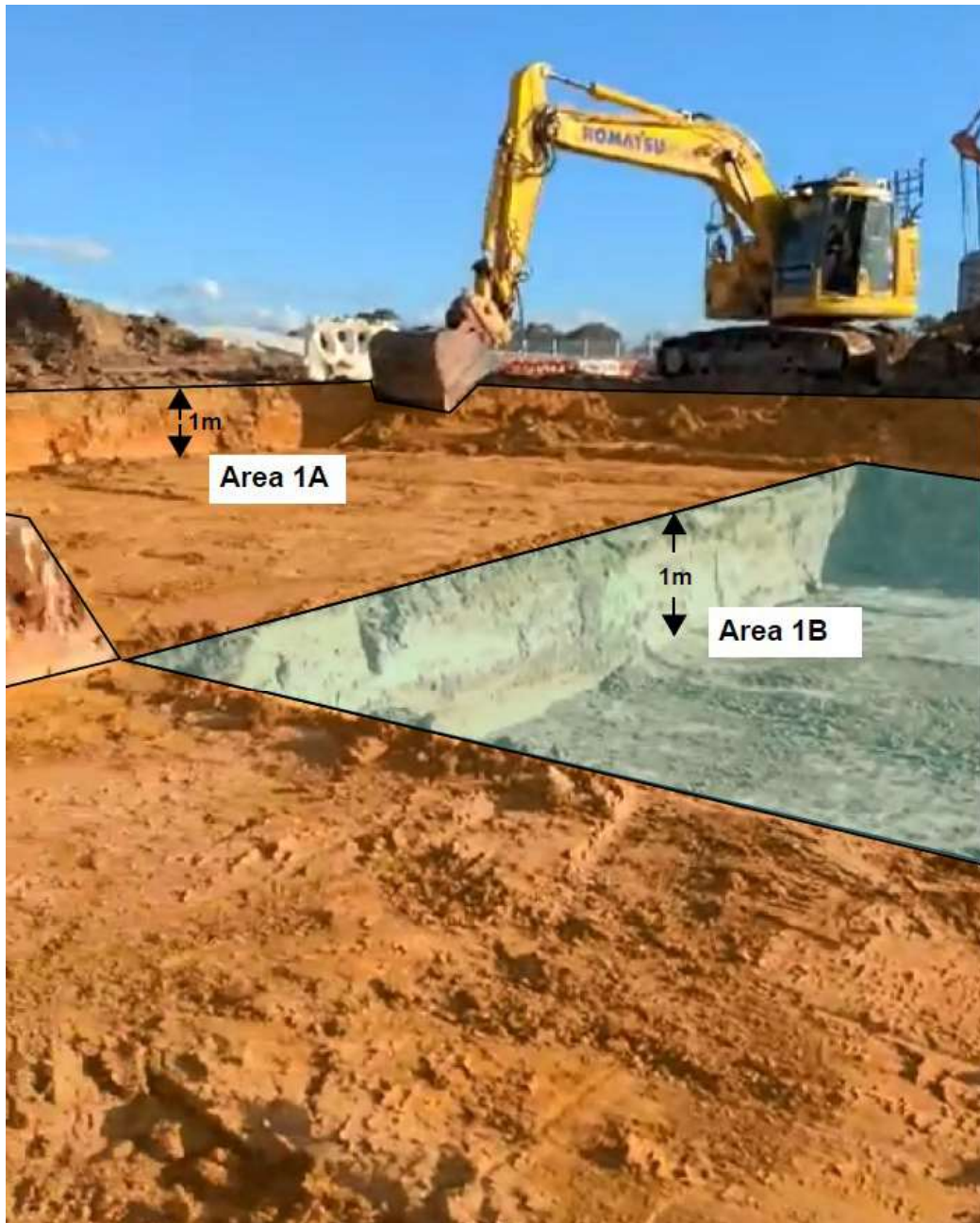
Excavation of PFAS Remediation Area 1A and 1B 1 June 2023
