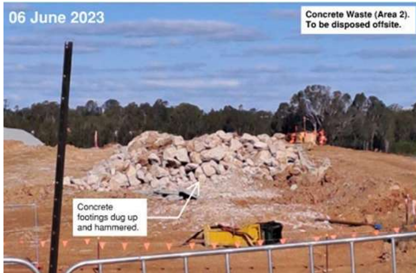
Figure F: Concrete footings from for RAAF Receiving Station
