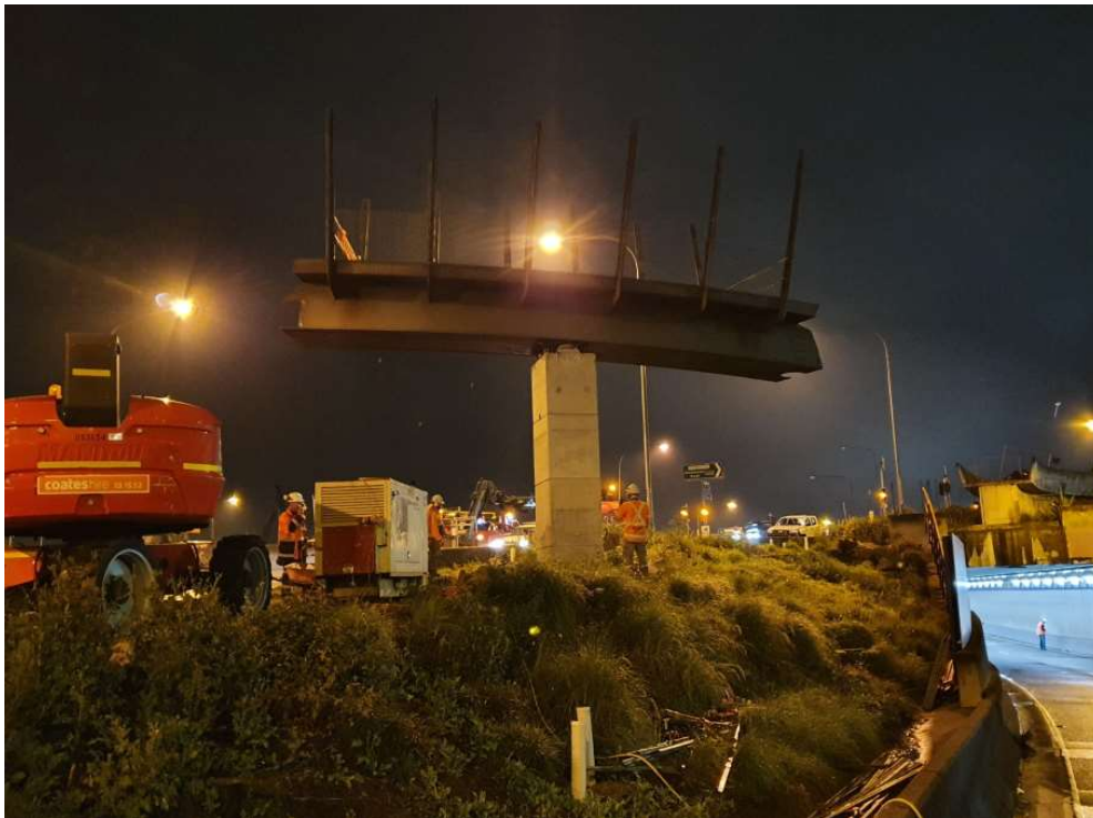
Figure 18- Leftover section above Pier 1
