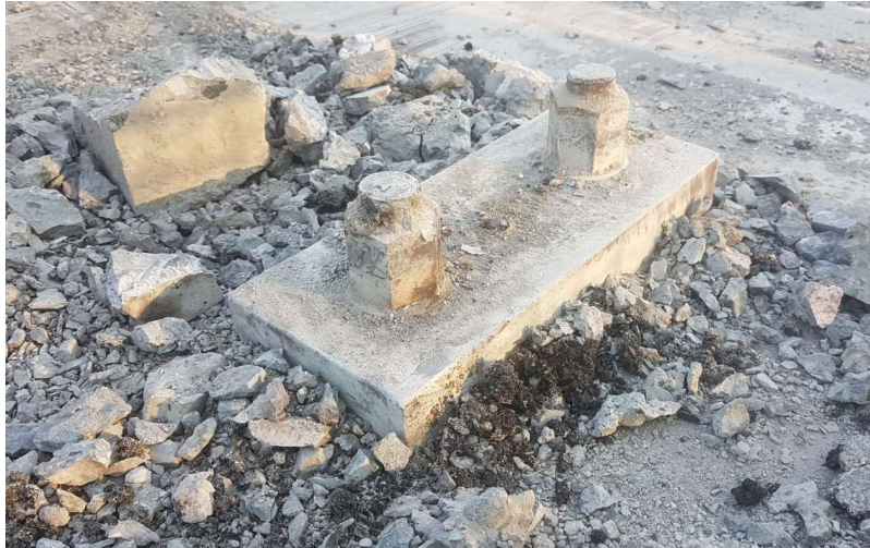
Figure 6- Exposed PT bar locking nuts
