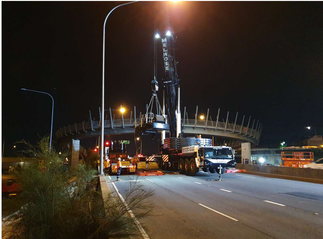
Figure 15- Mobile crane setting up on the Westbound side of Victoria Road
