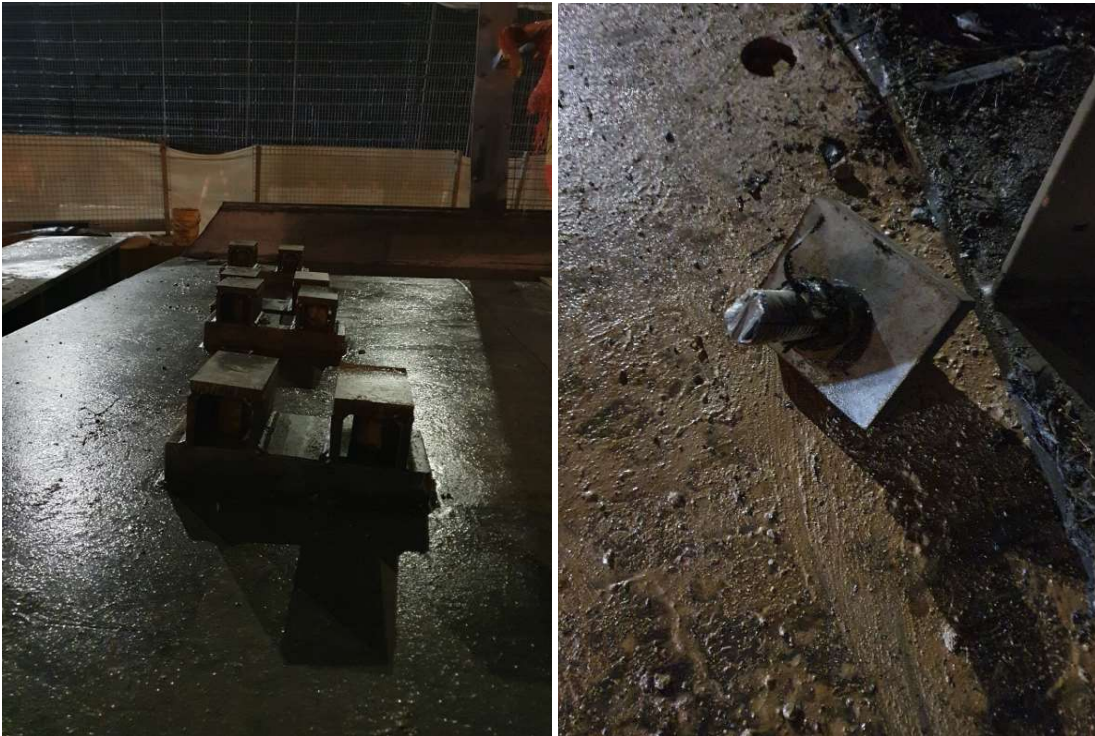
Figure 20- Inspection of stress bar brackets and cut stress bar
