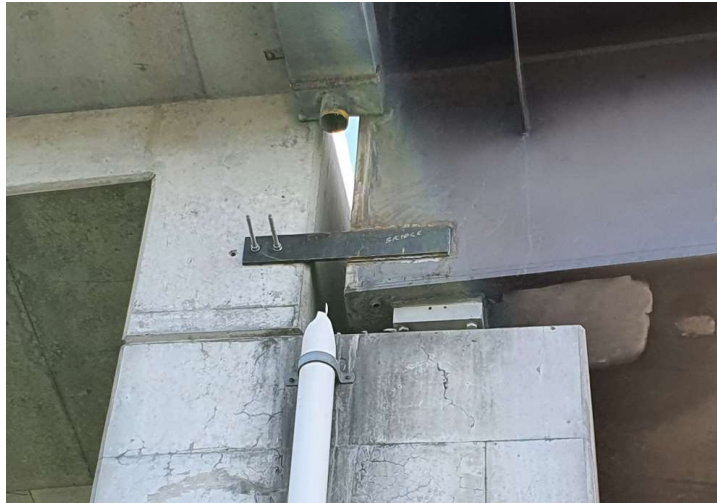
Figure 13- Temporary longitudinal restraint
