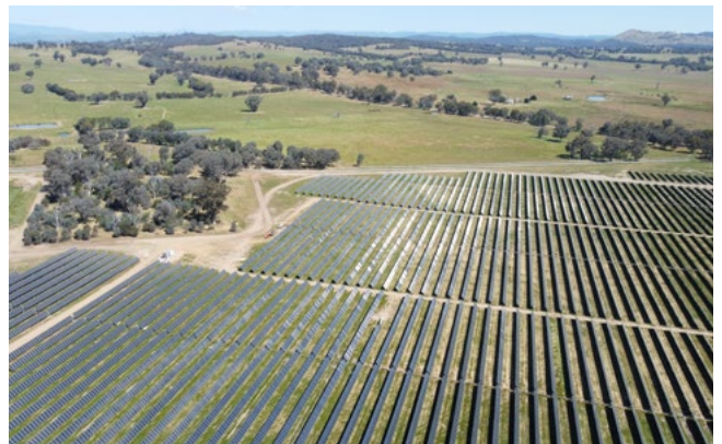
Solar panel installation completed in October 2023
