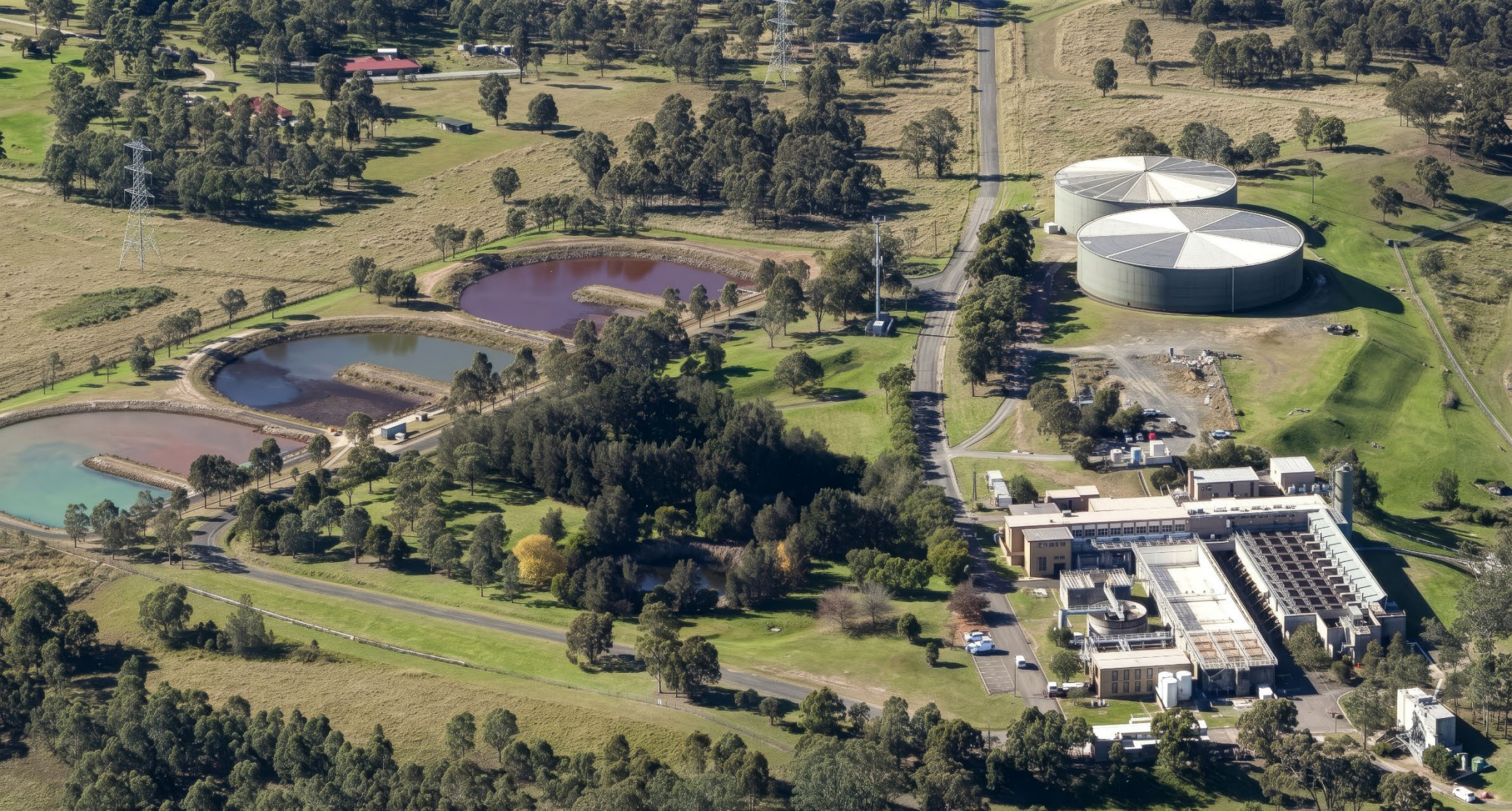
(Orchard Hills Water Filtration Plant, New South Wales)
