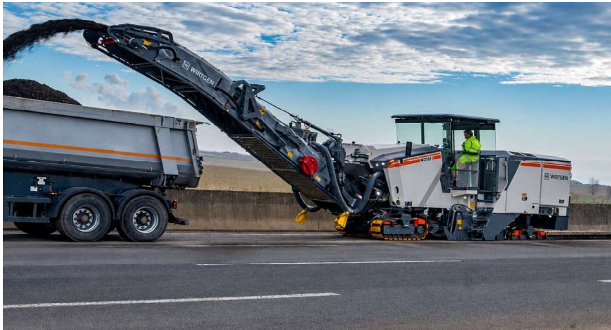
Collection of waste from milling operations.
