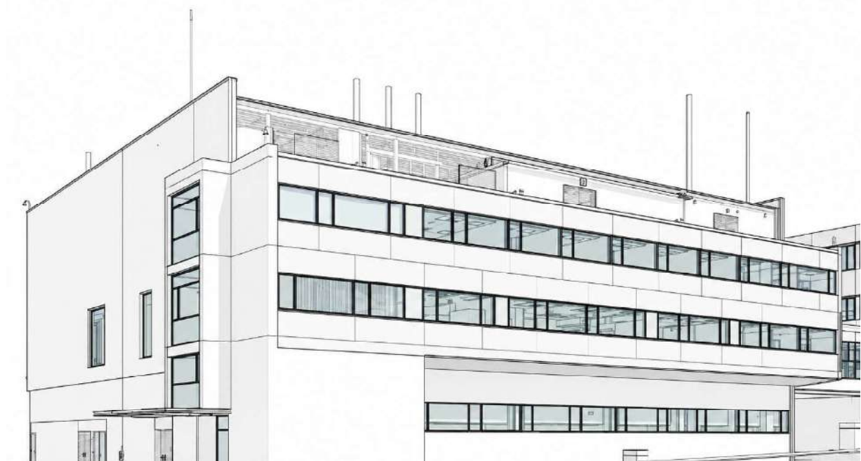
NCB4 facilities in Majadahonda.
