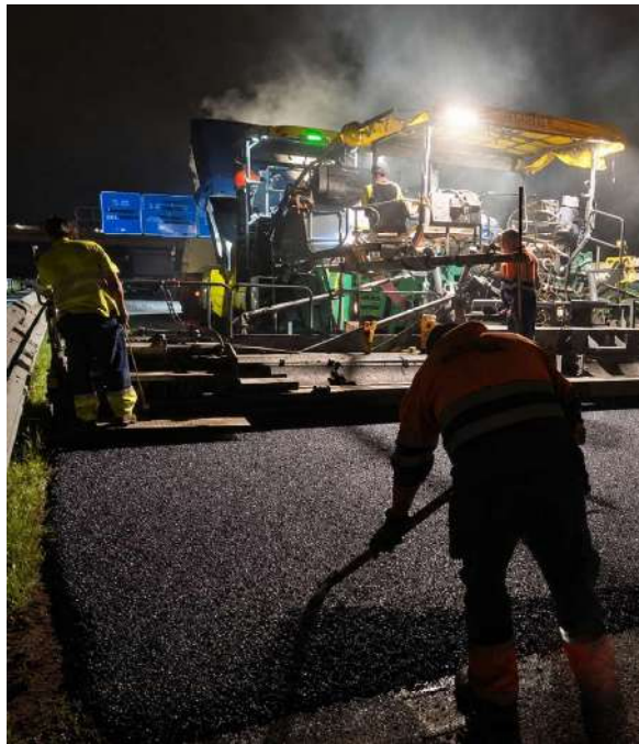
PA-16 paving on the trial section.
