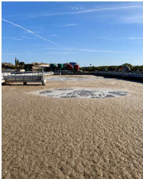
TOP: Previous situation — biological reactor with foam across practically the entire oxic zone, even preventing normal reactor aeration from being seen.
