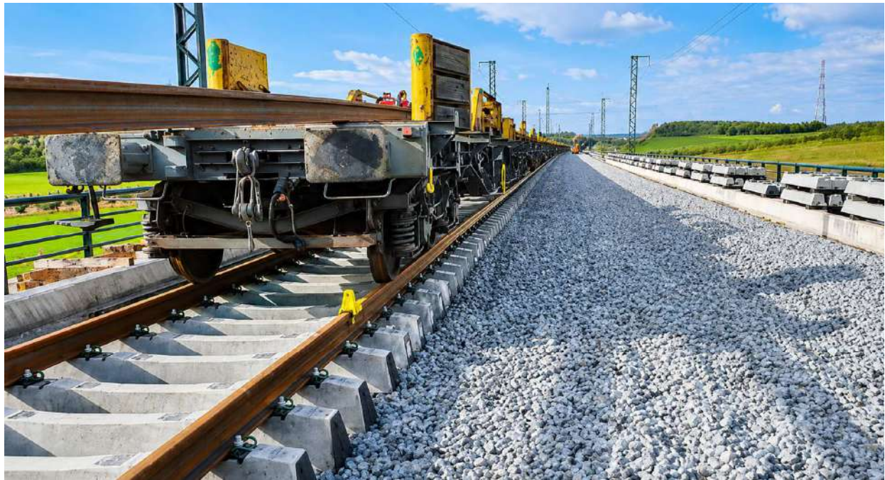
Spreading on railway trackbed.
