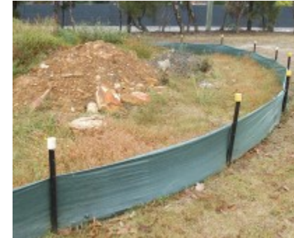
Install sediment control around spoil storage sites
