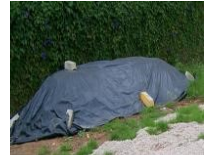
Store contaminated spoil on plastic or in a designated plastic lined receptacle and cover with plastic
