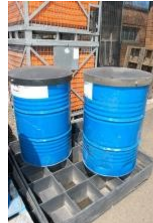
Drums on a portable bund
