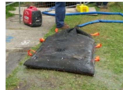
If discharge is cloudy/ turbid consider use of a dewatering bag
