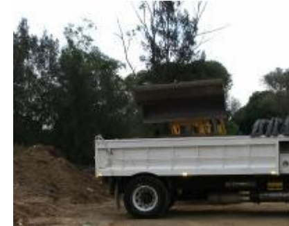
Obtain disposal dockets for each load of spoil disposed of at a licensed waste facility
