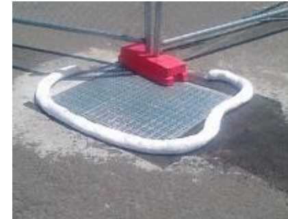
When responding to a spill, focus on protecting stormwater drains.
