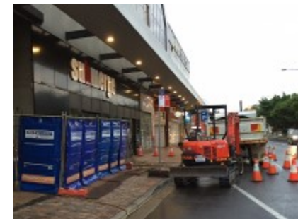
Temporary noise barriers installed to minimise out of hours noise impacts.
