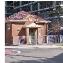
Heritage listed distribution substation
