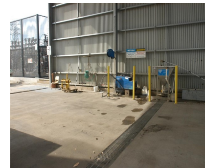
Vehicle wash bay— pressure hoses are to be used to limit water use. Do not leave hoses on unattended.
