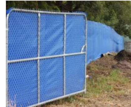
Attach dust barriers to fences of construction sites where required
