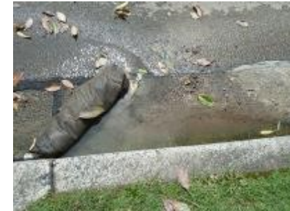
Sandbags/ gravel socks should be placed in gutters when dewatering to capture sediment
