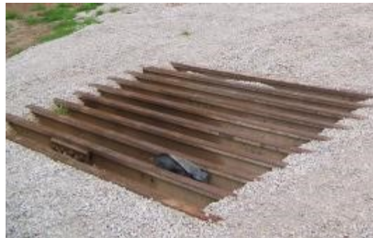
Install cattle grids and gravel beds at the site exit point
