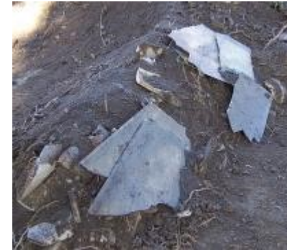
An example of asbestos contaminated soil
