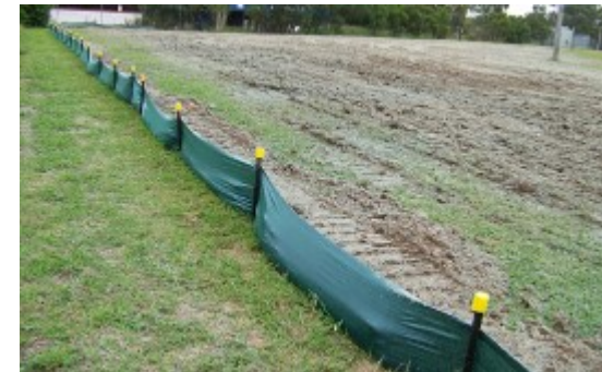
Spray grass and seeding can be used to stabilise a work site
