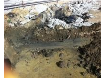
Discolouration of soils is a sign of potential contamination
