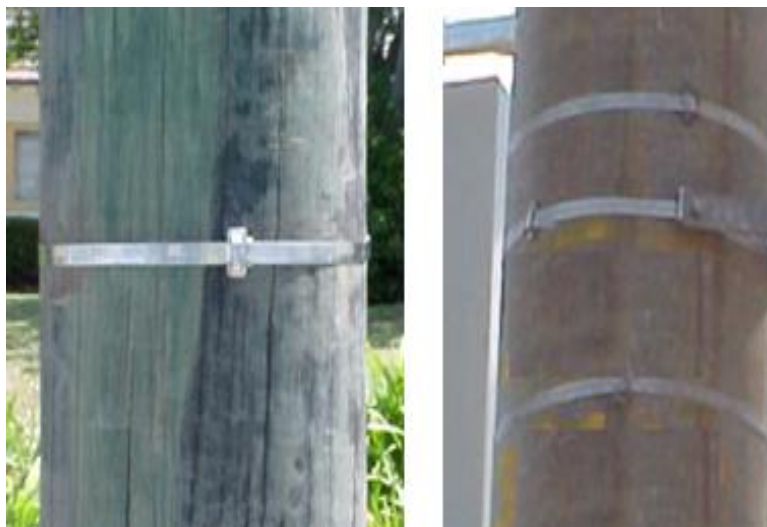
Figure 9 : Acceptable steel banding
