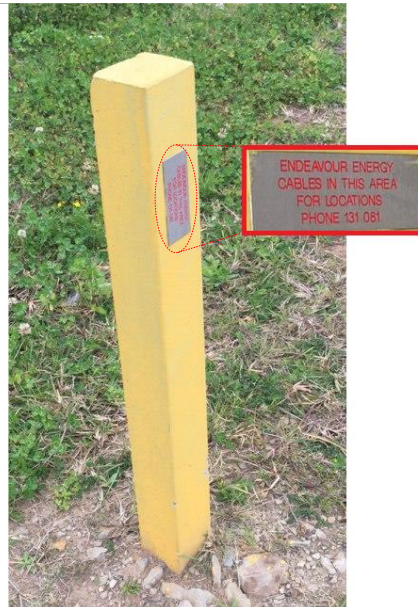
Figure 1: Typical cable route marker
