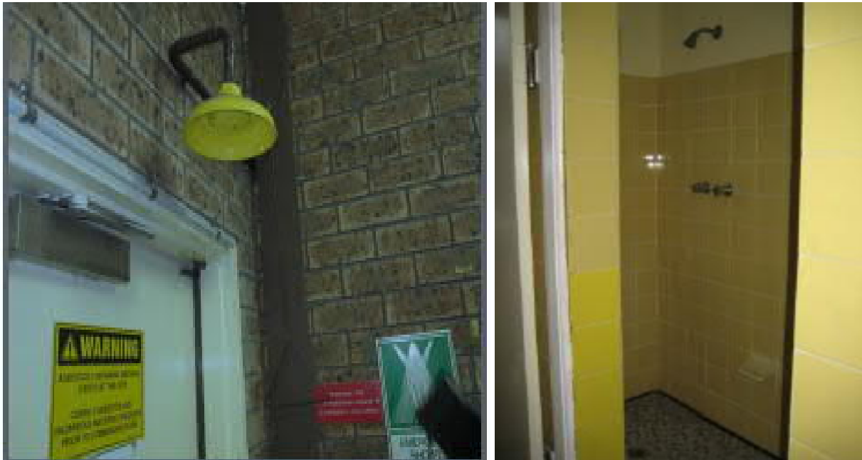
Example 2: Wet area inside substation building-N connectivity requirement determined by risk assessment
