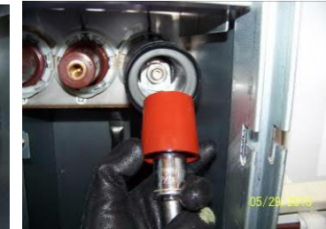
Figure 5 above right: The installation of the insulating (back) plug.
