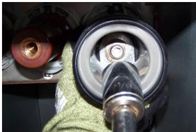
Figure 3 and 4 above left and centre: The securing washer and nut installed.
