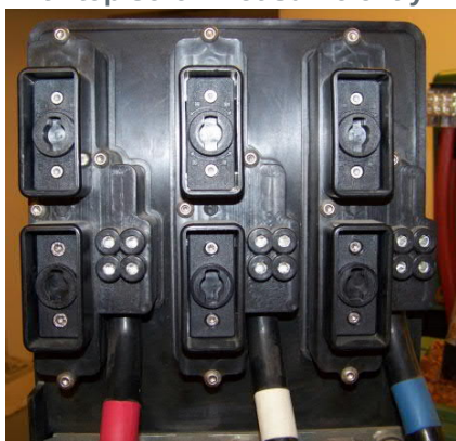
Figure 3: All links firmly locked into position during cable connection.
