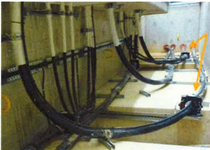
Cable screen earth conductor passed back through CBCT before bonding to earth.
