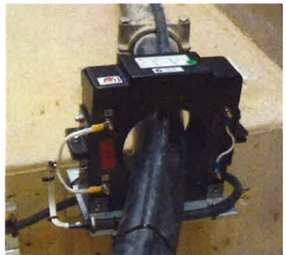
Cable screen earth conductor passed back through CBCT before bonding to earth.
