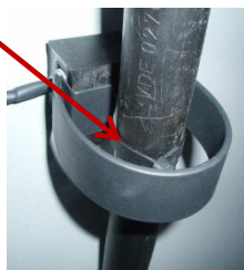
Figure 4-Close CT loop, ensure cable is in centre of loop
