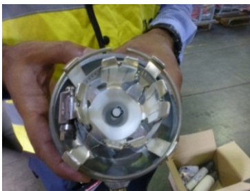
Figure 4 - Fuse holder with plunger
