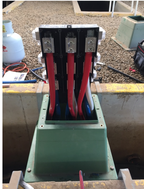
Figure 3 - New 3-link termination cable layout (horizontal phases)
