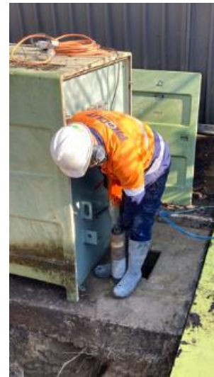
Fig. 2 Core hole drilling
