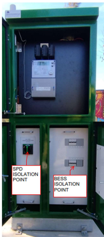
Figure 4 – LV Switchboard
