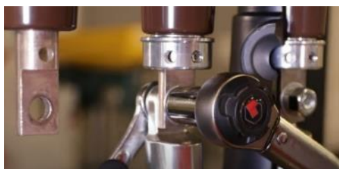
Fig. 5 Tightening cable lug with a torque wrench
