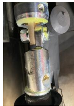
Fig. 4 Good connection of B & A phase
