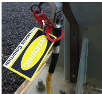
Figure 15 – Example locking mechanisms
