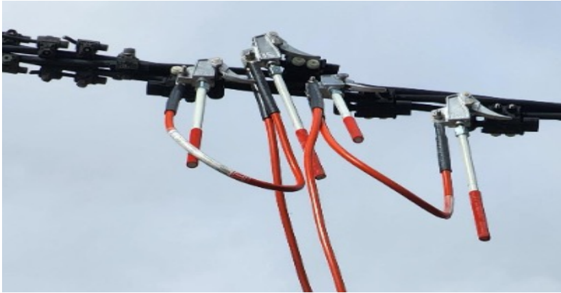
Figure 26 – Example application to overhead ABC mains
