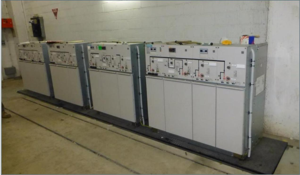
FIGURE 31 – Image of a Complex Distribution Substation's HV switchgear
