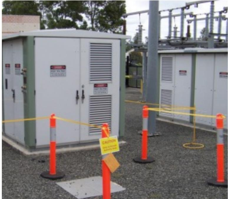
Figure 13 – Barrier “in” method for the erection of a barrier in a substation
