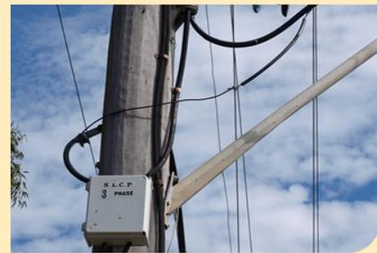
For work on pilot cables where the conductors are to remain unbroken and the cable will not be placed under mechanical stress, then the work may be carried out using live low voltage working procedures without the need to isolate the feeder or individual services within the cable.
