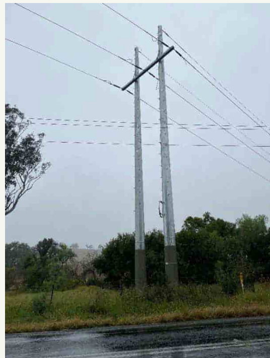
Image 10: View of steel power poles of the same type to be installed new as part of the proposed works.
