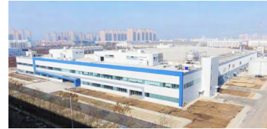
2015 Completed a semi-conductor assembly facility project for Micron in Xi'an.
