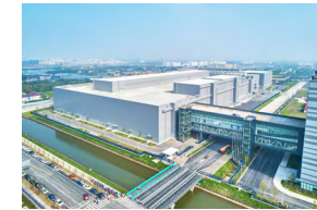
2019 Successfully completed a 300mm advanced production line 45 days ahead of schedule for HLMC.
