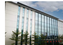
2016 Successfully delivered a data center project to Huawei and awarded "Excellent Project Team".
