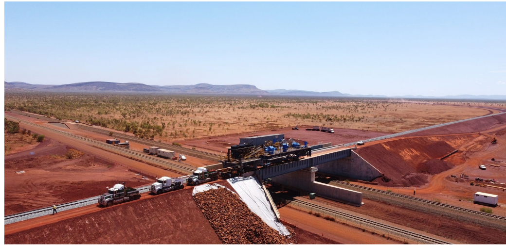
Eliwana rail bridge
