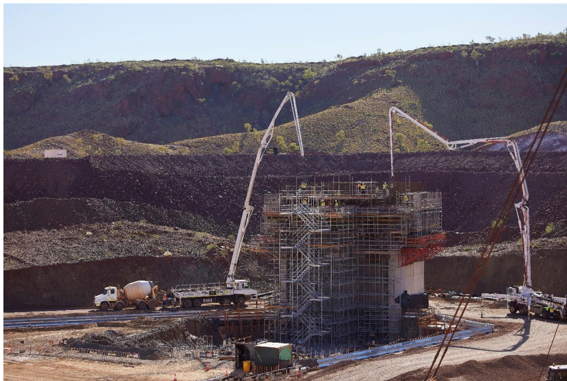
Construction of primary crusher
