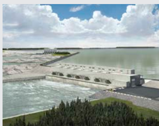
Keyask Hydroelectric Generation Project
